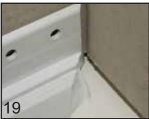
**19** Install the remaining strips in a similar manner. Before locating the remaining strips in position, butter Sealux-N slightly proud over the mitre cuts to ensure the Sealux-N fuses across meeting strips.
