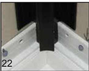
**22** The internal wall panel corner profile and outer edge profiles should be notched to overlap the bottom seal strip up-stand.
