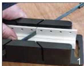
1. Screw the mitre box to a working surface. In a three sided installation, the middle strip will have two mitre cuts and be installed first. Strips with one mitre cut should be initially left a little longer than required - for now, when dry fitted into position they can be trimmed to the exact length as defined by the strip end mark on the wall.
