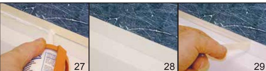
**27/29** When all the wall panels are installed, 'pressure apply' Sealux-N into the joint formed between the wall panel and adjacent strip. Rub up the Sealux-N smooth and carefully remove the masking tape.
