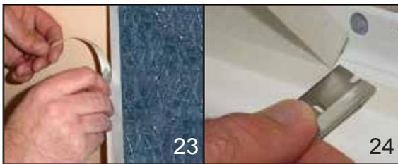
**23/24** To prevent smearing with Sealux-N, apply masking tape over bottom outer face of the wall panel and outside face of the strip outer leg. Trim the over hang flush with a bohemian blade. Do not extend masking tape over wall panel surfaces being covered by corner and edge trims.
