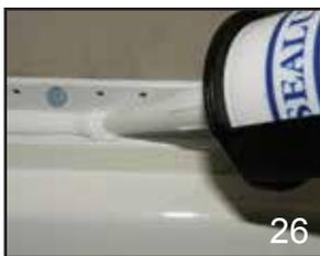
**26** Prepare the wall panel for fixing in accordance with the instructions. Immediately prior to mounting each panel on the respective strip, apply a continuous line of Sealux-N into the strip channel formed between the strip up-stand and wall panel support leg. Offer the wall panel simultaneously against the wall and onto the strip. Fix the wall panel to wall ensuring it is located parallel with the strip.
