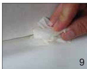
9 Clean the ledge using the alcohol wipes. Dry fit the strips in position once again and apply 3 removable marks or 3 pieces of masking tape on the ledge to define the proposed outside boundary of each strip when fitted. Remove the spatula and end caps from the end cap card.
