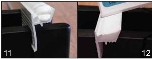
**11/12** Rest the nozzle on the strip and apply a 400 millimeter line of Sealux-N into the strip. Flush fill the Sealux-N across the strip resting the spatula on the outside strip edge and the inner leg. You can add Sealux-N or redistribute the Sealux-N as required with the spatula. Continue this process in 400 millimeter intervals until the strip is complete.
