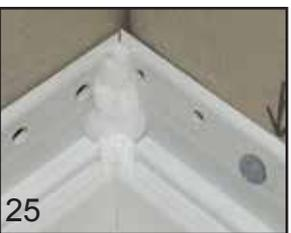
**25** Apply Sealux-N to fill notched holes and extend over the meeting strip up-stands at corner joints.
