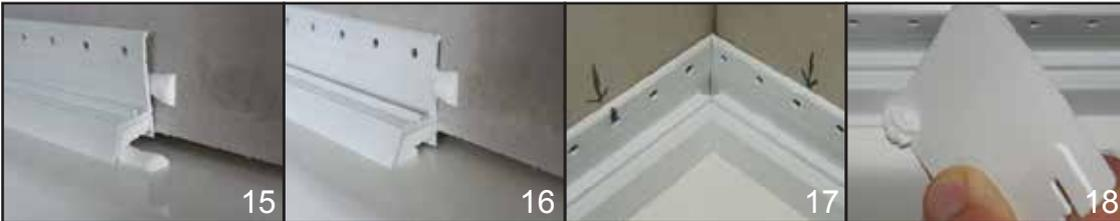
**15/18** Offer the strip over the joint and rotate it into position, in the process fusing the Sealux-N in the strip with the Sealux-N on the ledge to form a watertight seal. The position of this first strip should then be fine tuned by dry fitting the adjoining strips and ensuring all joints meet symmetrically. Remove any surplus Sealux-N located outside the strip end with the spatula.
