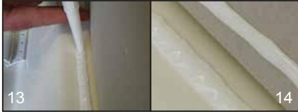
**13/14** With your finger under the nozzle for support and your fingertip against the wall as guide, lay an 8mm line of Sealux-N on the ledge so that outer edge is no more than 20 mm from wall or just inside the 3 marks previously applied in step 9. Apply a light line of 'high grab' polymer adhesive on the wall approximately 15 millimeter over the ledge.
